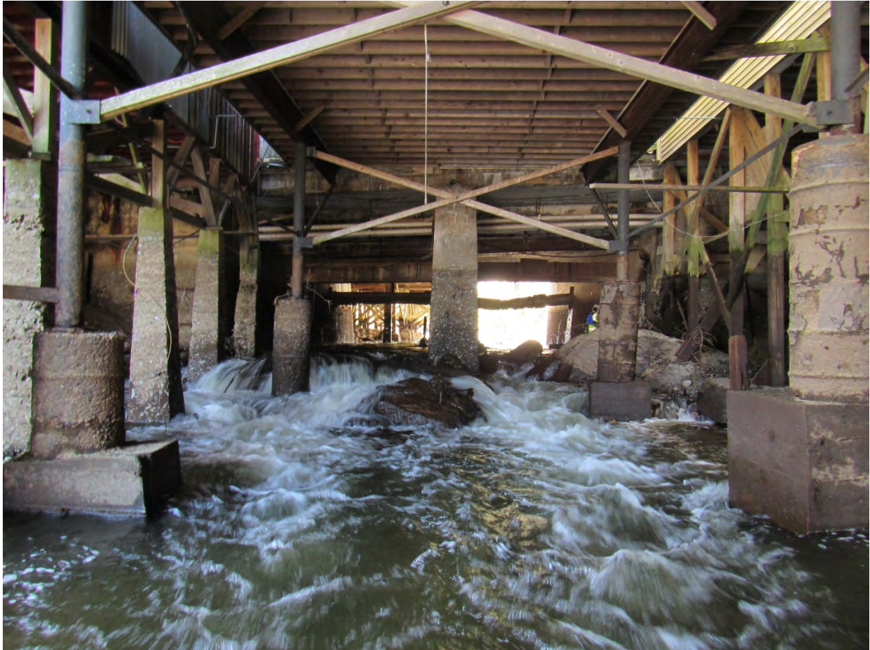
Figure 28. View upstream at Main Street bridge in drawn down condition, May 8, 2018. Hydraulic drop at downstream bridge opening in center of photo. Stain lines apparent on posts indicate normal pool elevation.
