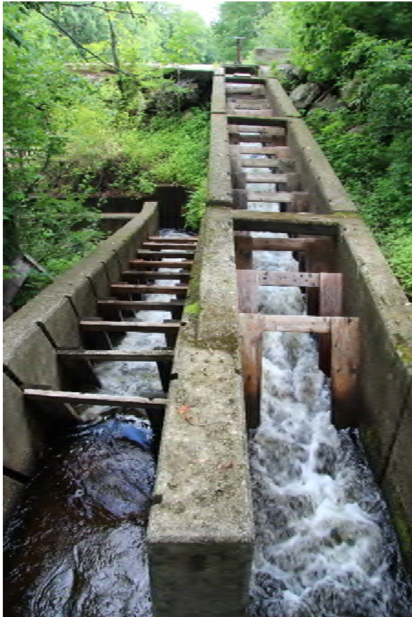
Figure 93. Example of a Denil fishway.
