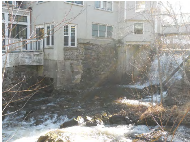
12) Knowlton Street Dam (south spillway) and 51 Mechanic Street
