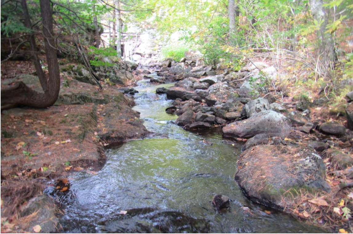
Figure 54. Looking upstream at the channel flowing from the West Dam. Steep bedrock forms the right bank of the channel.
