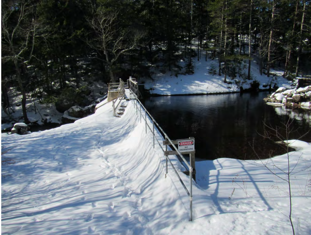
Figure 57. The East Dam in 2019.
