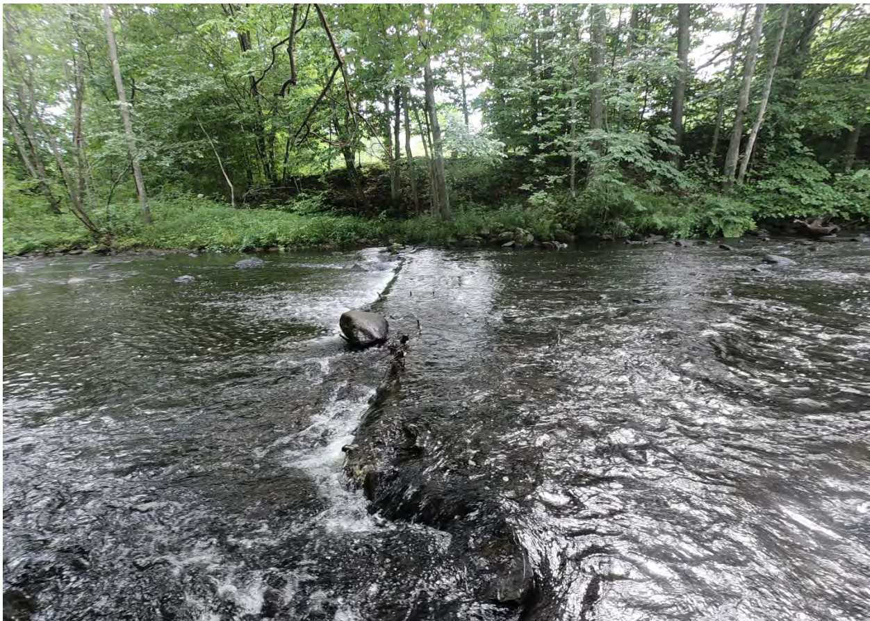
Figure 47. The remnants of a wooden crib dam approximately 330 feet downstream of the Powder Mill Dam.
