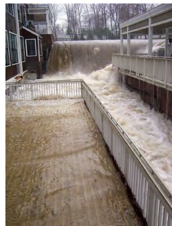
24) Knox Mill Dam – High water overtopping 32 Mechanic Street deck and impacting the upstream end of 40 Washington Street deck (Photo courtesy of Alison McKellar, Town of Camden)
