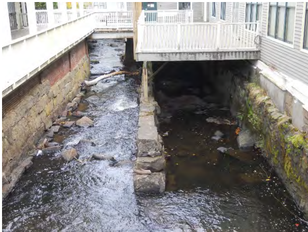
27) 40 Washington Street (left), 32 Mechanic Street (right) and connecting decks – Stone foundations
