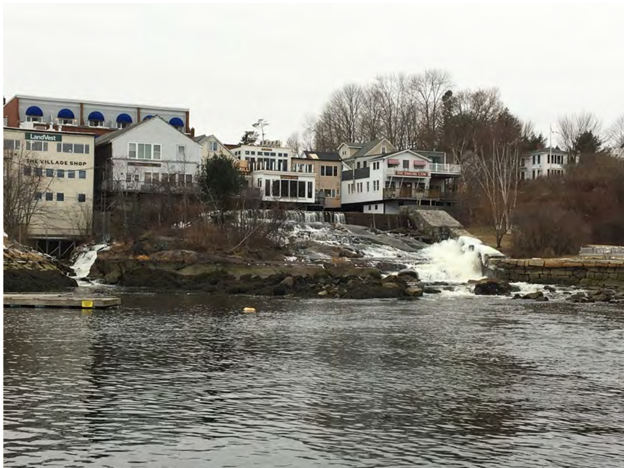
Figure 25. The outlet of the Megunticook River from Camden Harbor. Montgomery Dam sits atop the bedrock. The Harbor Park is to the right of the photo and the Public Landing is to the left.
