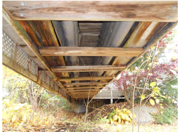
20) Knowlton Street Dam – Underside of pedestrian bridge with utility conduits
