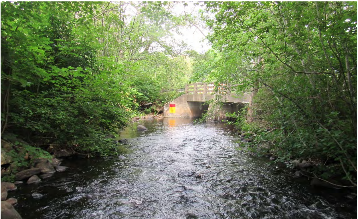
Figure 44. Looking downstream at the Rawson Street crossing.
