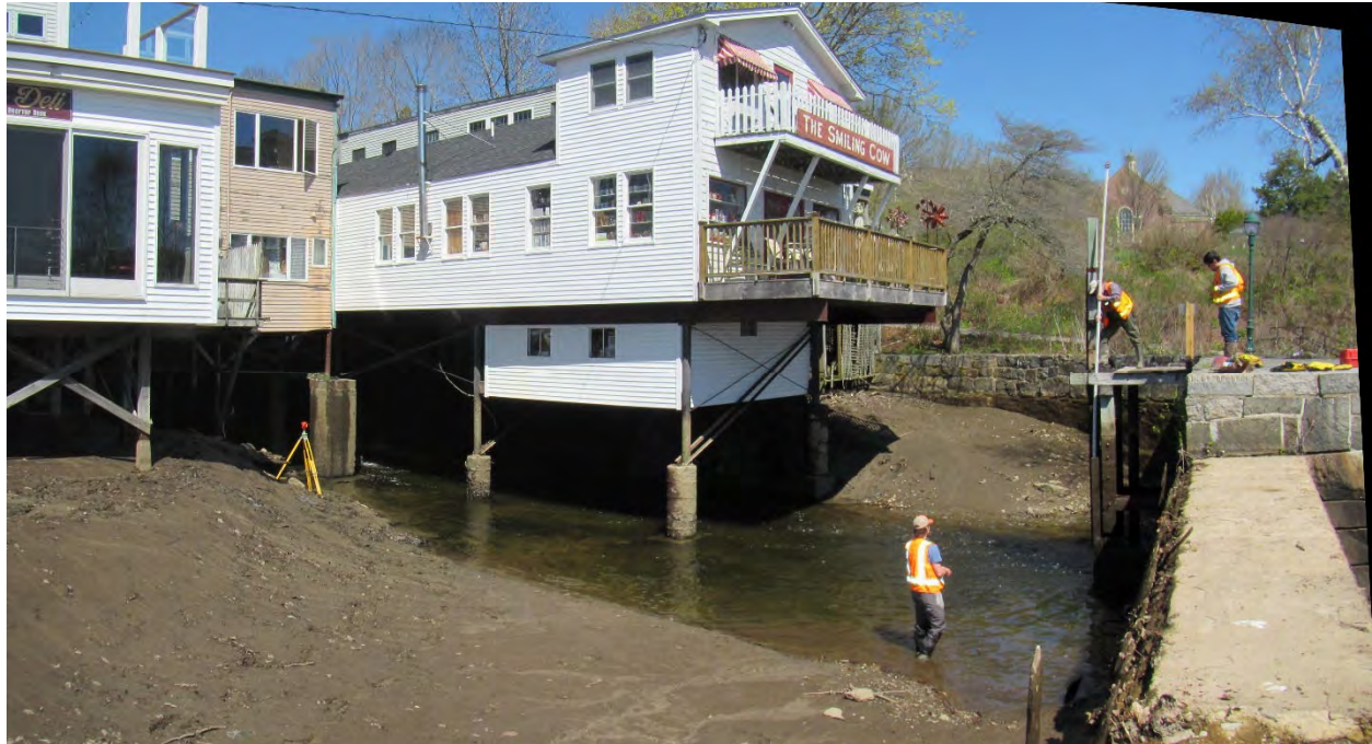
Figure 26. View of lower impoundment and north end of spillway in drawn down condition, May 8, 2018.
