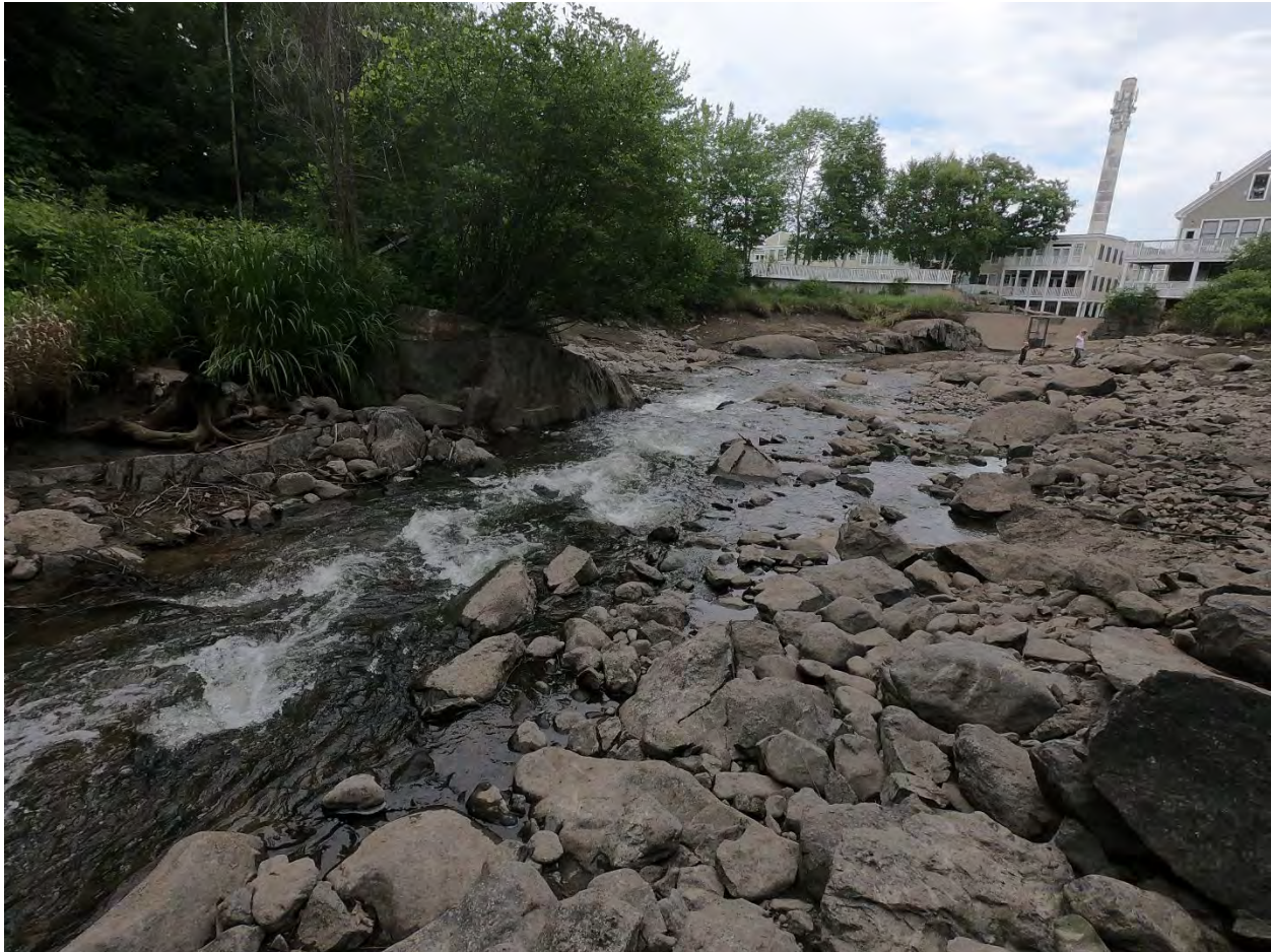
Figure 34. Looking downstream at the Knox Mill impoundment in a drawn down condition. The coarse bed material and relatively modest amount of impounded sediment are evident.
