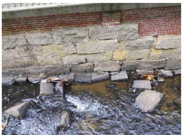
30) 32 Mechanic Street – Minor repairs are needed; dam removal may change but not significantly worsen existing conditions
