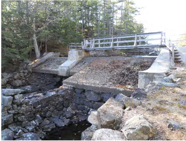
1) Megunticook Lake Dam East
