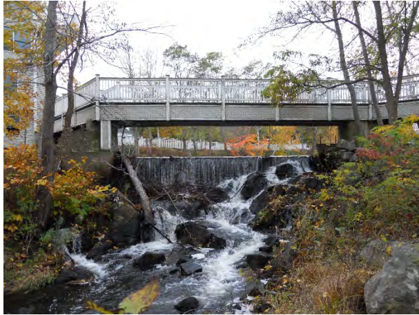
19) Knowlton Street Dam (north spillway) and pedestrian bridge to 2 Knowlton Street
