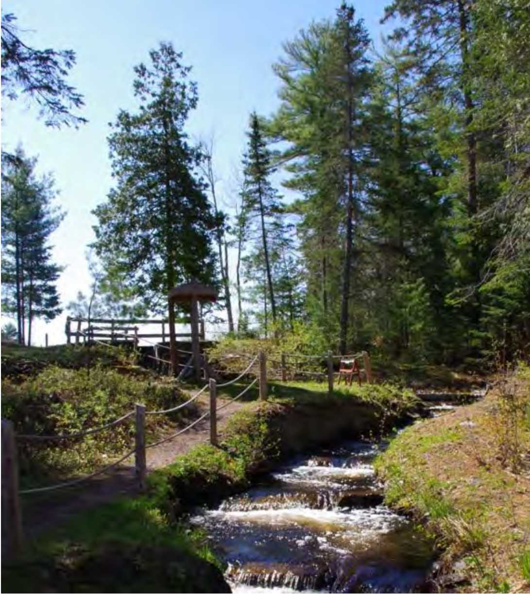
Figure 92. Pool and weir fishway at Blackman Stream (photo credit: Maine Sea Grant).
