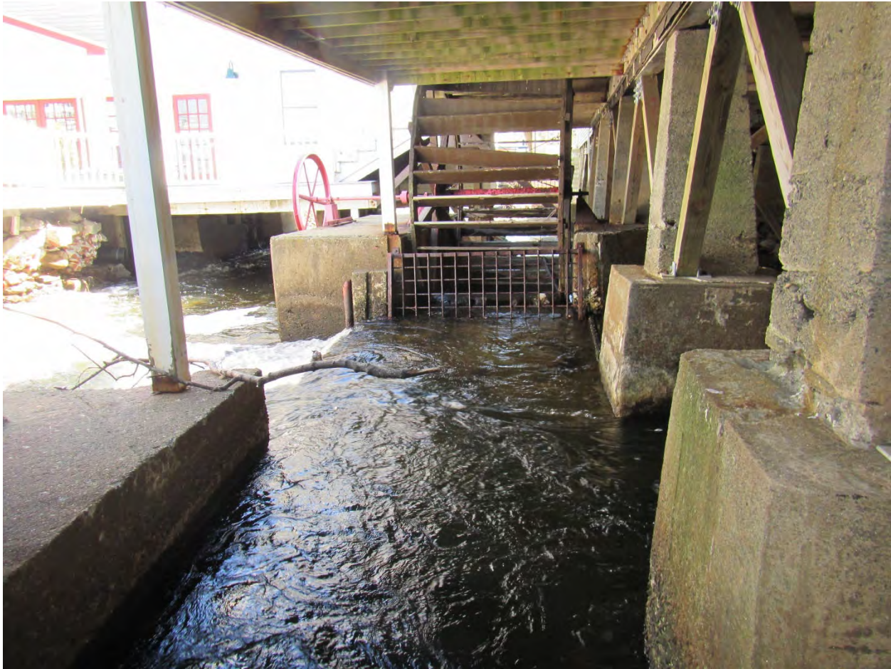
Figure 5. Relict water wheel and weirs beneath the former Brewster Shirt Factory.
