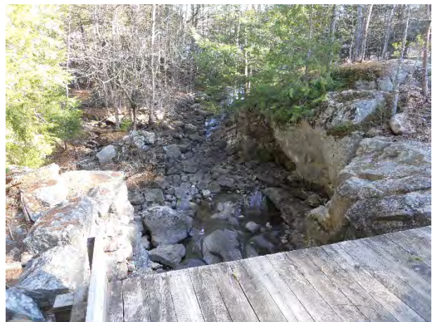
6) Megunticook Lake Dam West – View downstream
