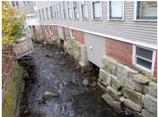
28) 36 Washington Street (left) and 32 Mechanic Street (right) – Stone foundations
