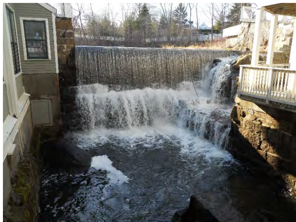
23) Knox Mill Dam, 32 Mechanic Street (left) and 40 Washington Street (right) – View upstream
