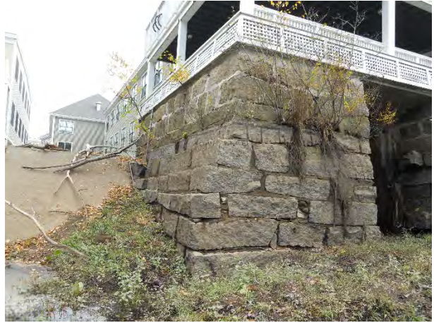
26) 32 Mechanic Street (NW corner) – Lowered water condition
