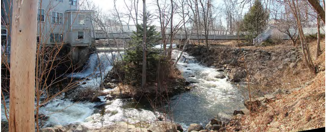
Figure 38. Split flow downstream of Knowlton Street dam, with assisted living facility on river right.
