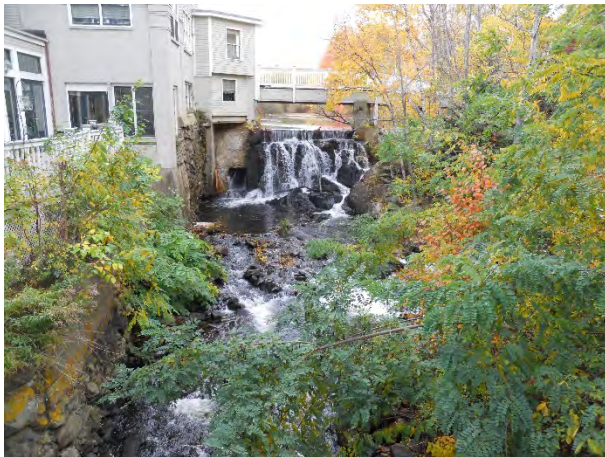
15) Knowlton Street Dam (south spillway) and 51 Mechanic Street
