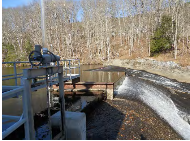
8) Seabright Dam spillway
