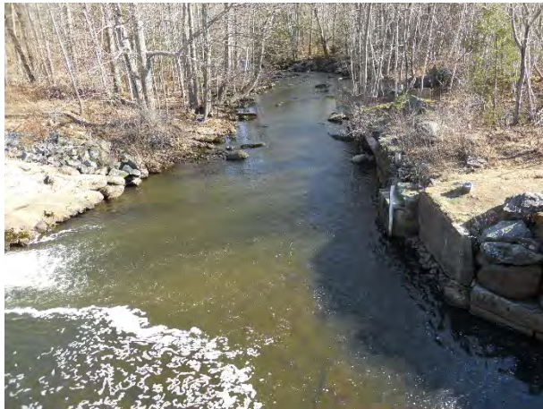
9) Seabright Dam – View downstream
