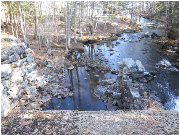
3) Megunticook Lake Dam East – View downstream
