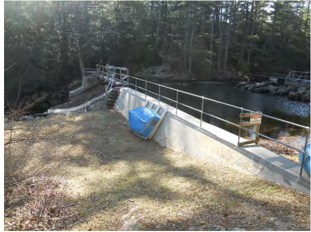
2) Megunticook Lake Dam East
