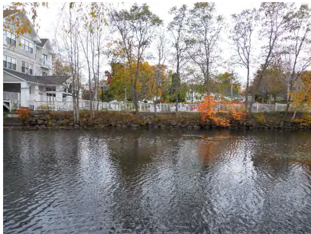
21) 51 Mechanic Street and parking lot – gravity retaining wall along shore
