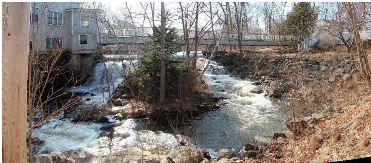
Figure 97. Composite photo of the existing side channel (right side of photo) through which fish passage could be attained under a dam removal scenario at Knowlton Street Dam.
