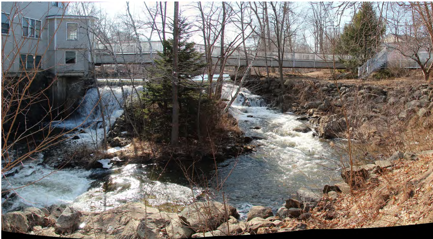
Figure 110. Ground-level composite image of the Knowlton Street dam site, March 2021.
