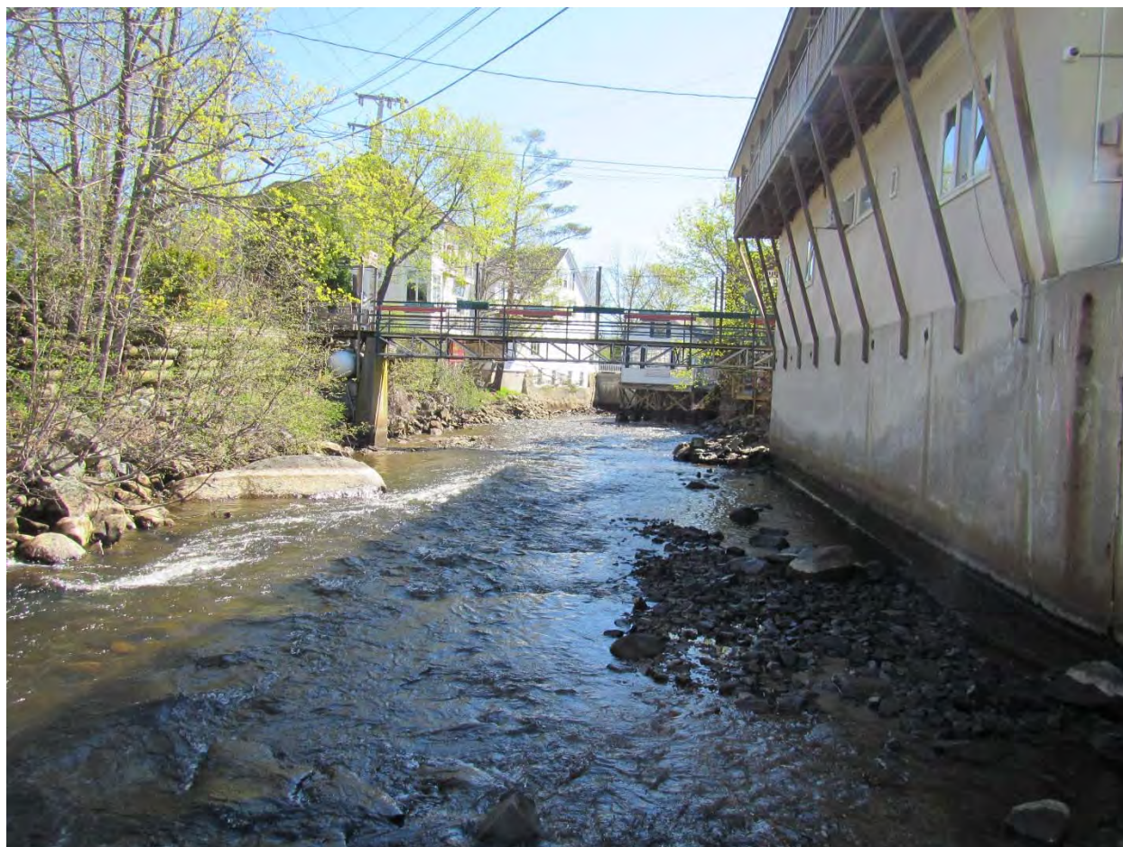
Figure 22. View of upper impoundment looking downstream from Brewster building in drawn down condition, May 8, 2018. Stain lines on large boulder at left, and concrete wall at right indicate normal pool elevation. The ground to the left of the channel is comprised of urban fill.
