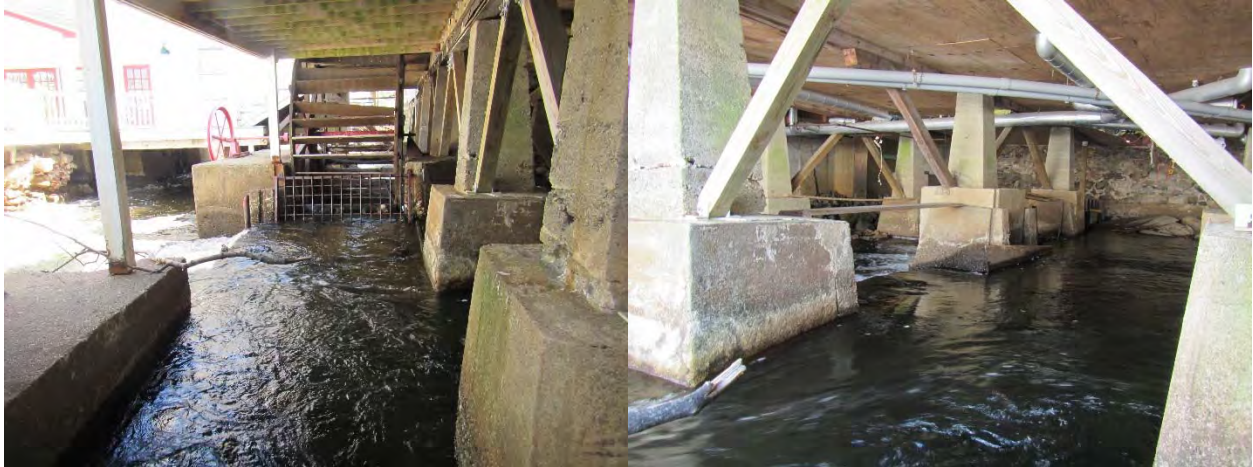
Figure 28. Looking downstream beneath Brewster building, May 8, 2018. Relict water wheels and weirs between pier footings visible in images.
