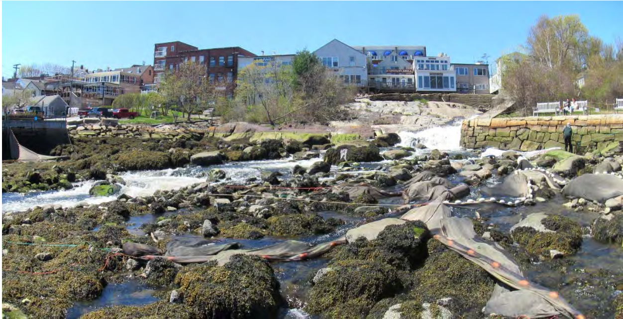
Figure 10. View from head of harbor looking upstream at ledge outcrop and Montgomery dam, May 8, 2018. The seawall is shown in the right foreground.
