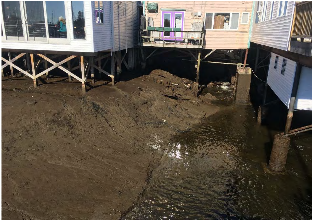
Figure 30. The impoundment with the water level drawn down. A modest volume of fine-grained sediment is trapped behind the dam. May 8, 2018. Relict tank location is immediately below and several feet downstream of the purple French doors in the image.
