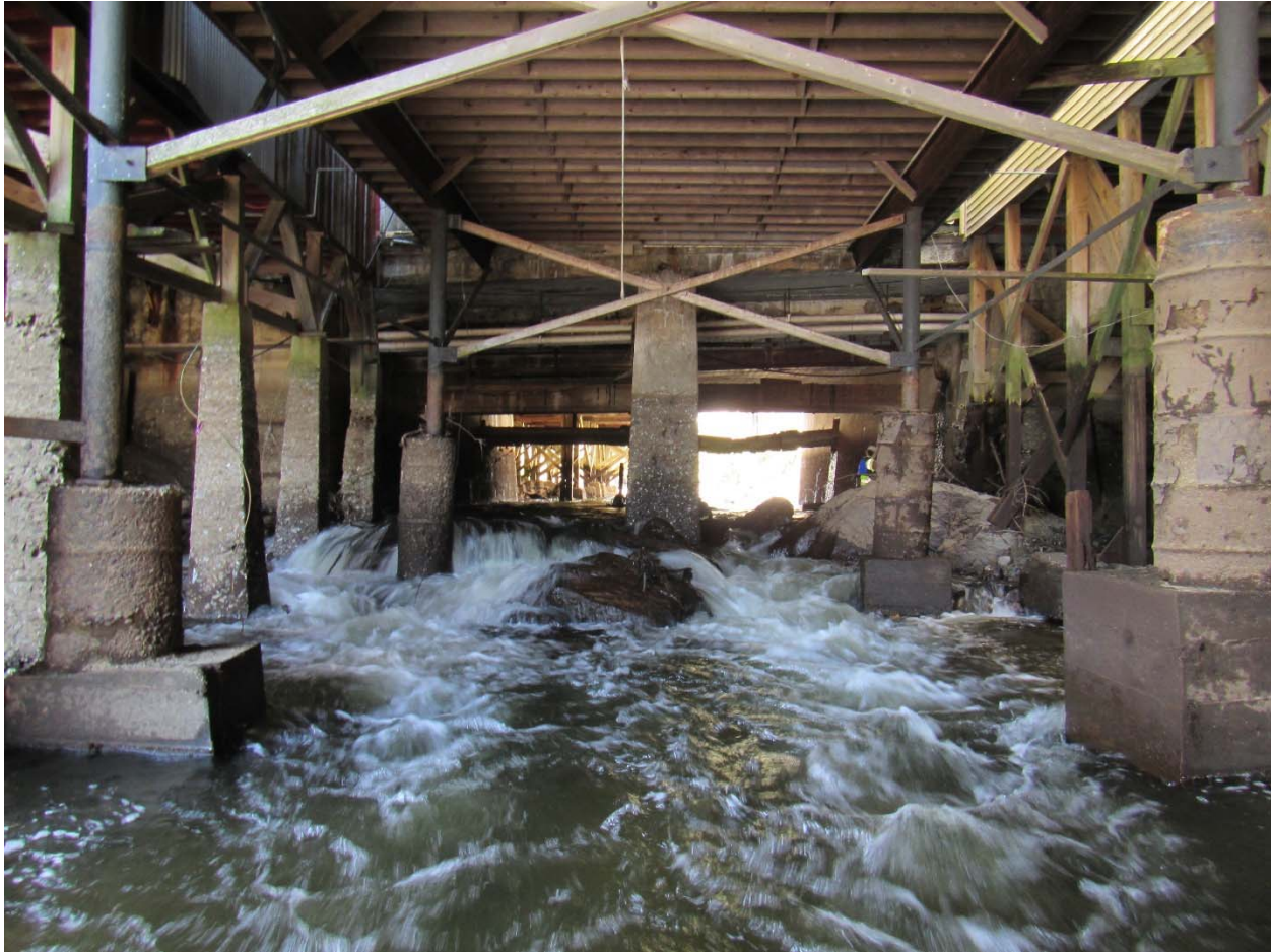
Figure 26. View upstream at Main Street bridge in drawn down condition, May 8, 2018. Hydraulic drop at downstream bridge opening in center of photo. Stain lines apparent on posts indicate normal pool elevation.
