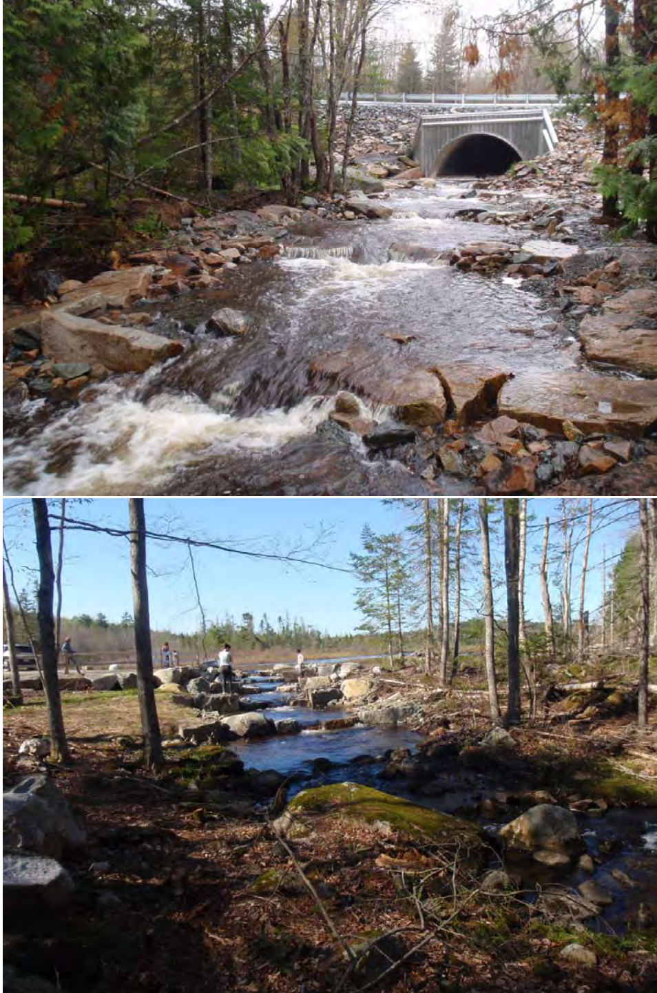
Figure 43. Examples of constructed nature-like fish passage (photo credits: Matt Bernier).
