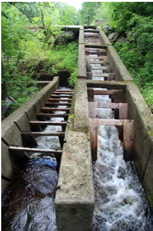
Figure 46. Example of a Denil fishway.
