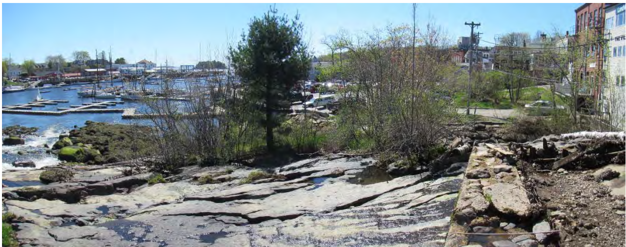
Figure 13. View of south end of spillway and ledge outcrop, May 8, 2018.
