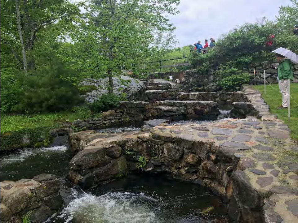
Figure 44. Pool and weir fishway at Damariscotta Mills.
